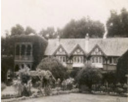
B0062 Murndal Homestead Murndal Rd Hamilton
