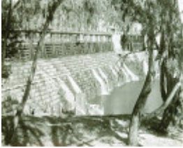
B0897 Goulburn Weir Complex Nagambie
