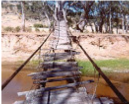
B5279 Suspension Bridge
