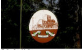
The Euroa Butter & Ice Factory. The oldest and one of three surviving butter manufacturing sites in Victoria. A number one rated in 1910, it has been listed by the State. Plans for the first three-story building were quickly approved and construction for 1910 started. By 1911 it was open for business. The building is a prime historic site and is the only one of its kind in the region. It is the only one of its kind in the region.
