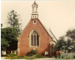
B1829 St Malachy's Catholic Church 363 High St Nagambie
