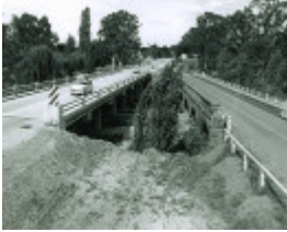
B1743 Hughes Bridge Hume Hwy Avenel
