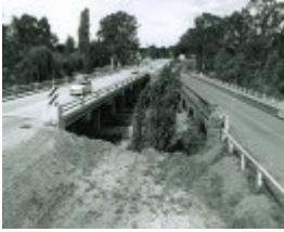
B1743 Hughes Bridge Hume Hwy Avenel
