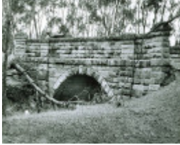
B1592 Pranjip Creek Bridge
