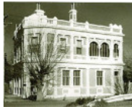
B5170 Former Colonial Bank
