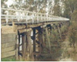
B6849 Mitchellstown Bridge
