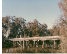
B6849 Mitchellstown Bridge
