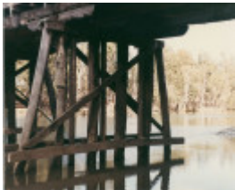
B6849 Mitchellstown Bridge piers
