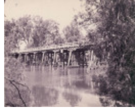
B6849 Mitchellstown Bridge
