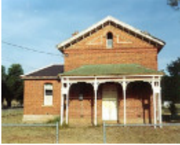
B1538 Fmr Court House Queen St Avenel
