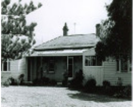
B1619 Aitkenside Cochrane's Road
