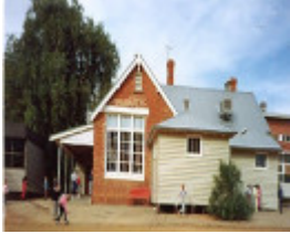
B5642 Former Primary School No 1142
