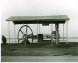
B1643 Cannie Ridge Irrigation Pump Foreshore Lake Boga
