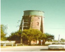
B4866 Water Tower, Monash Drive
