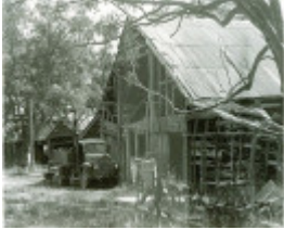
B4559 Stable Building Noorongong
