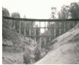
B6949 Darbyshire Hill Bridges
