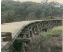
B6949 Darbyshire Hill No. 1 Bridge
