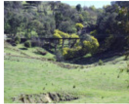
B6949 Darbyshire Hill No. 1 Bridge
