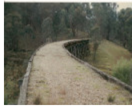
B6949 Darbyshire Hill No.1 Bridge
