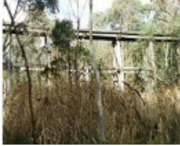
b6951 Darbyshire Creek No 2 Bridge
