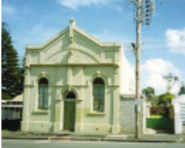
B6204 Former Premier Butter Factory
