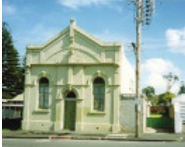
B6204 Former Premier Butter Factory
