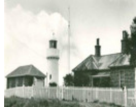
B1336 Lighthouse Complex
