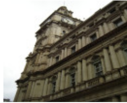
h00903 gpo bourke street2
