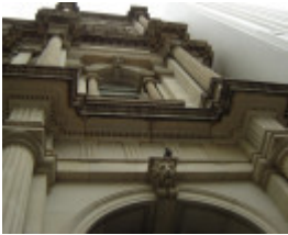
h00903 gpo bourke street
