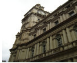
h00903 gpo bourke street2
