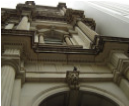
h00903 gpo bourke street
