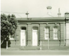
B4526 Offices 67 - 69 Kepler Street
