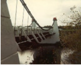
B1706 Wollaston Suspension Bridge Warrnambool
