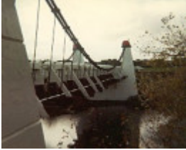
B1706 Wollaston Suspension Bridge Warrnambool
