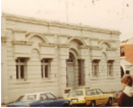
B4978 RSL Building
