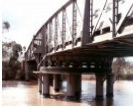
B2379 Swing Bridge
