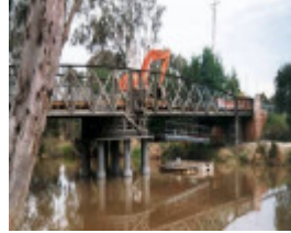
B2379 Swing Bridge Being Renovated
