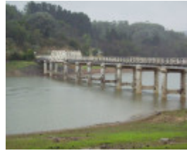
B7097 Glenmaggie Truss Bridge
