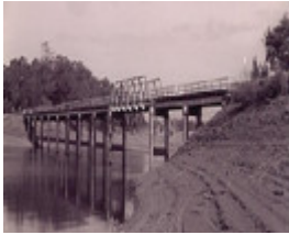
B7097 Glenmaggie Truss Bridge
