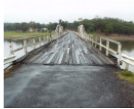
B7097 Glenmaggie Truss Bridge
