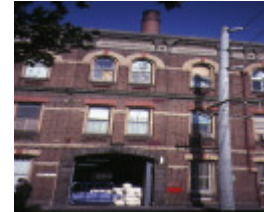
former denton hat mills nicholson street abbotsford delivery entrance
