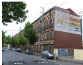
FORMER DENTON HAT MILLS SOHE 2008
