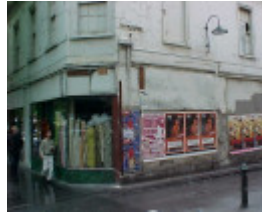
H00435 jobs warehouse bourke street melbourne croseley's building oct01
