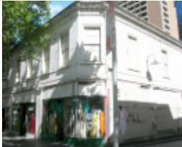
JOBS WAREHOUSE SOHE 2008
