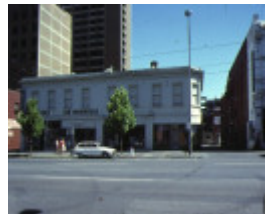
H00435 jobs warehouse bourke street melbourne croseley's building jan1979
