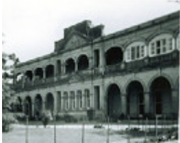
B2969 Kilmany Park Homestead
