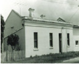
B1220 Fmr Bond Store 41 Wharf St Port Albert
