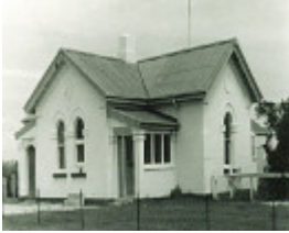
B2732 Post Office Wharf St Port Albert
