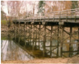
B6924 Wodonga Creek Bridge
