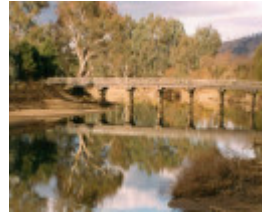
B6924 Wodonga Creek Bridge
