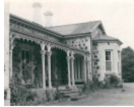
B2847 Benyeo Homestead Side View
