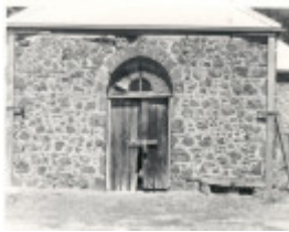
B2847 Benyeo Homestead Woolshed Fanlight
