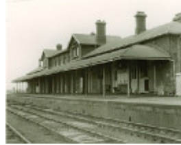
B2371 Railway Station Serviceton
