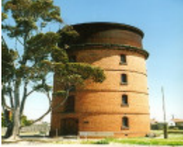
B2728 Water Tower Murtoa
