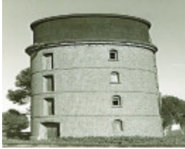
B2558 Water Tower
