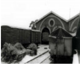
B3215 Railway Buildings
