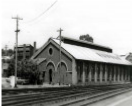
B3215 Railway Buildings
