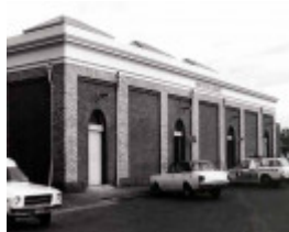
B3215 Railway Buildings
