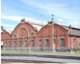
B3215 Railway Buildings
