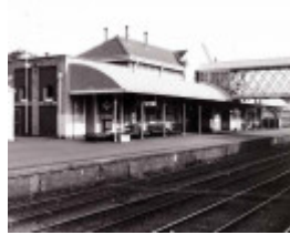
B3215 Railway Buildings
