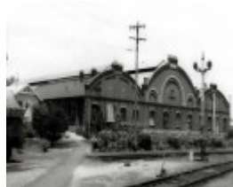
B3215 Railway Buildings
