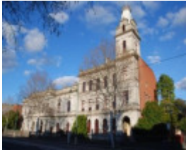
B5052 School of Mines Building - Group Classification
