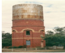
B5767 Water Tower
