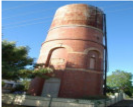
B5767 Water Tower
