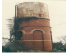
B5767 Water Tower
