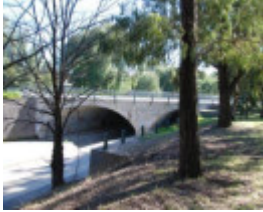
B7071 Weeroona Avenue Bridge
