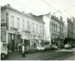
B7231 Bourke St East
