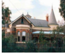
B7237 Hawthorn Grove Historic Precinct
