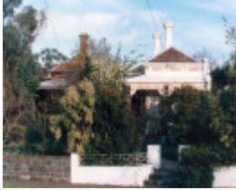
B7237 Hawthorn Grove Historic Precinct
