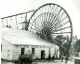
B4894 Gold Reefs Crushing Works
