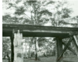
L10003 Rail Bridge Central Park
