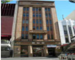
FORMER BANK OF NEW SOUTH WALES SOHE 2008
