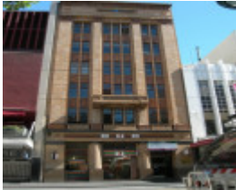
FORMER BANK OF NEW SOUTH WALES SOHE 2008
