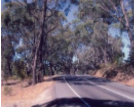
L10138 Pyrenees Highway
