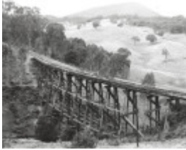
Cudgewa Line Trestle Bridge
