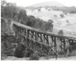
Cudgewa Line Trestle Bridge
