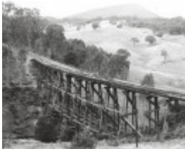
Cudgewa Line Trestle Bridge
