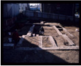
CAMP STREET PRECINCT EXCAVATION
