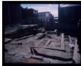
CAMP STREET PRECINCT EXCAVATION
