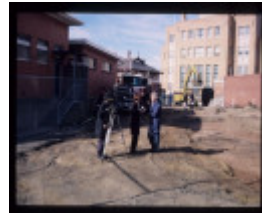
CAMP STREET PRECINCT EXCAVATION
