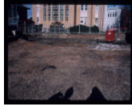
CAMP STREET PRECINCT EXCAVATION
