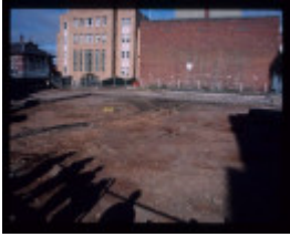
CAMP STREET PRECINCT EXCAVATION
