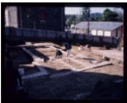
CAMP STREET PRECINCT EXCAVATION
