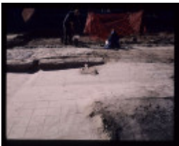
CAMP STREET PRECINCT EXCAVATION
