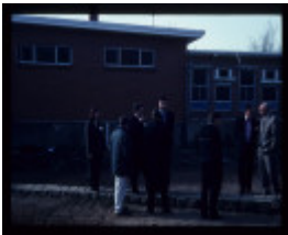
CAMP STREET PRECINCT EXCAVATION
