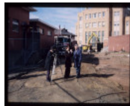
CAMP STREET PRECINCT EXCAVATION
