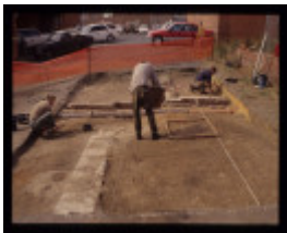
CAMP STREET PRECINCT EXCAVATION
