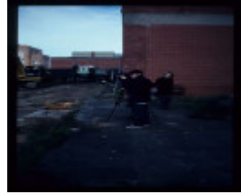
CAMP STREET PRECINCT EXCAVATION
