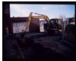
CAMP STREET PRECINCT EXCAVATION
