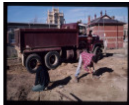
CAMP STREET PRECINCT EXCAVATION
