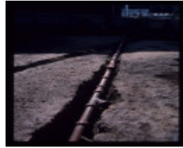
CAMP STREET PRECINCT EXCAVATION
