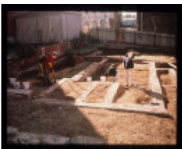
CAMP STREET PRECINCT EXCAVATION
