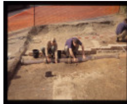
CAMP STREET PRECINCT EXCAVATION
