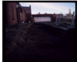
CAMP STREET PRECINCT EXCAVATION
