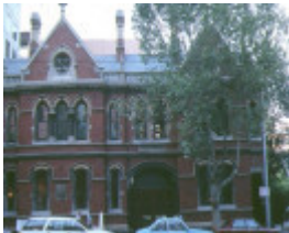
old bourke street west police station & cell blocks bourke street melbourne front elevation
