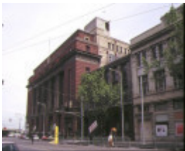
former mail exchange bourke street melbourne rear view
