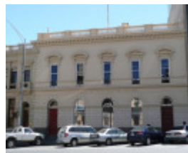
FORMER BANK OF NEW SOUTH WALES SOHE 2008
