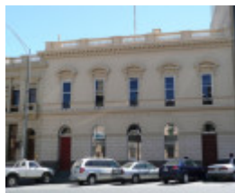
FORMER BANK OF NEW SOUTH WALES SOHE 2008
